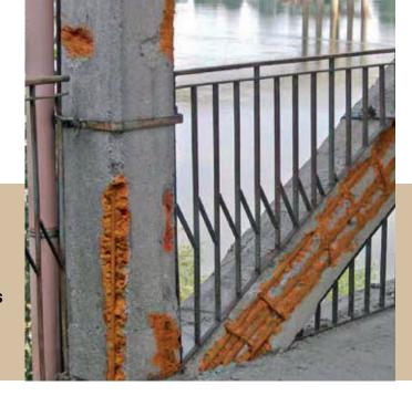
**PASSIVATING** is a one-component, reddish-colored mortar based on cementitious binders, synthetic resins, microsilica and special corrosion inhibiting additives
