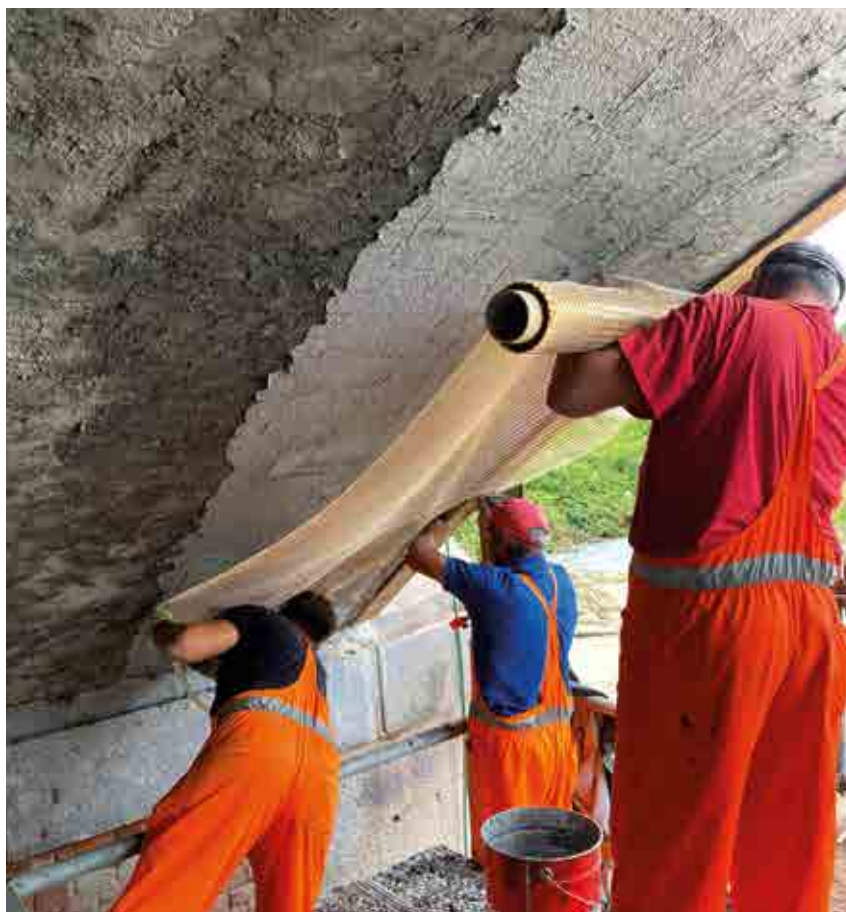
Securing and strengthening the Cavour Canal Bridge - Formigliana (VC) • FRCM structural strengthening system with PBO-MESH 22/22 and PBO-MESH 44 mesh, and MX-PBO Masonry inorganic matrix.
