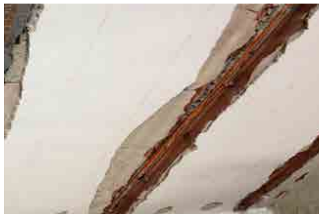
The first stage of the procedure involves removing the discontinuous parts of the joist in concrete and cleaning and passivating the concrete rebars .
