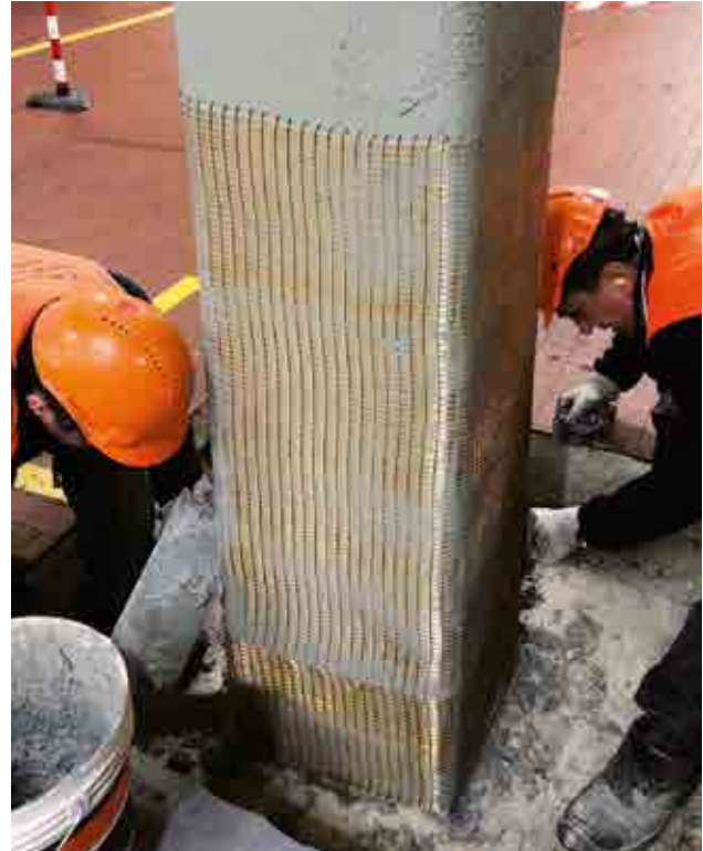
Shear strengthening and confinement of a column.
