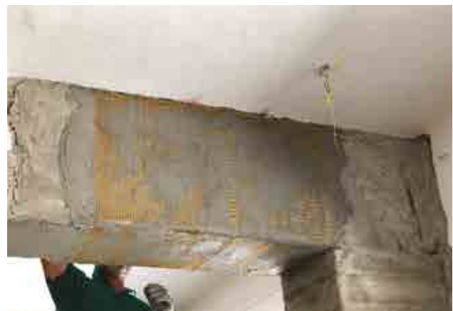
Shear strengthening.
