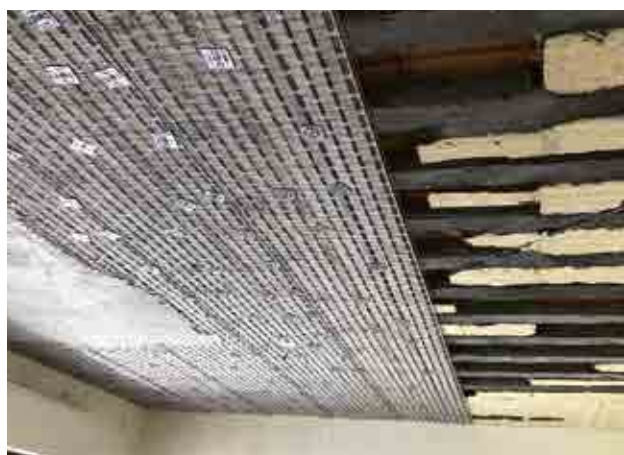
Applying the STUCANET ceiling anti-shatter system.
