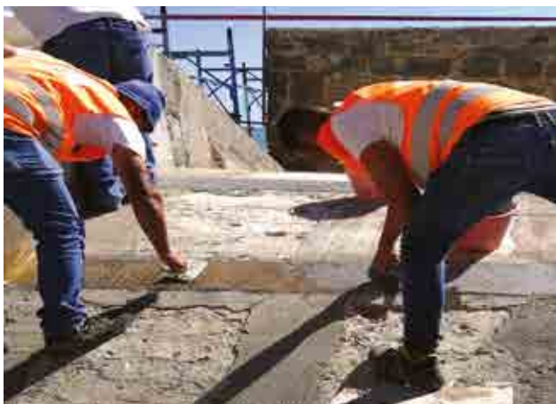
Strips in grid layout extrados (upper side) strengthening.
