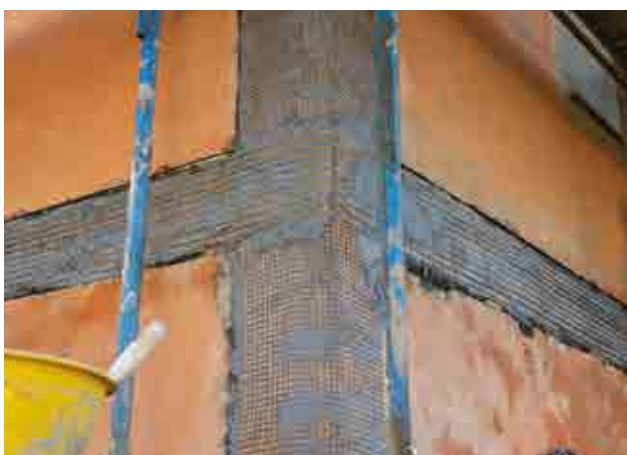
Strengthening of masonry corners and floor edge beams.
