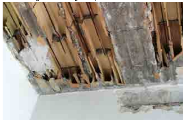
Shatter and falling of ceiling fragments caused by water leaks, resulting in expansion of the brickwork , and accelerated ageing of the intrados (lower side) of the slab, coupled with corrosive oxidation of the joist concrete rebars .
