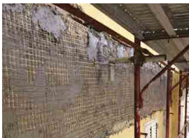
Applying the FRCM system.
