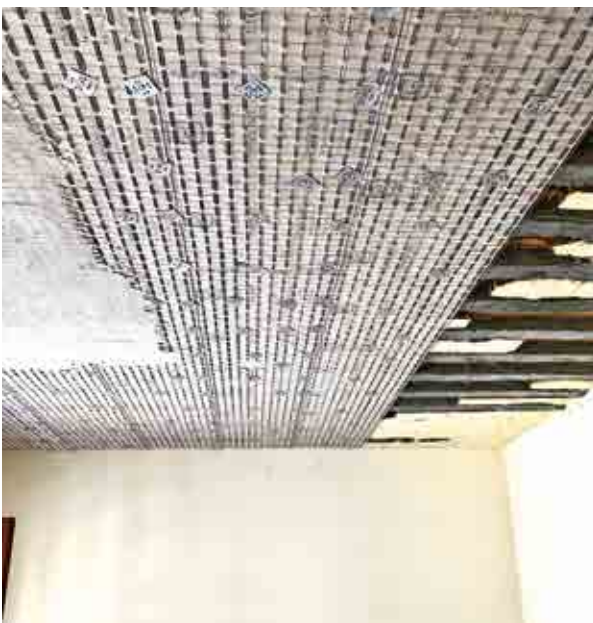
STUCANET system installed
