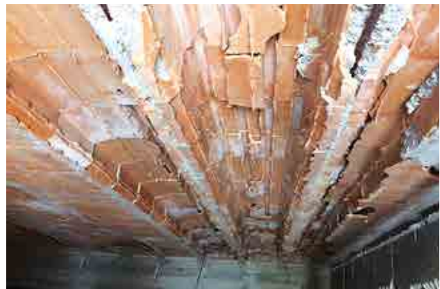
Hazardousness of shatter and falling of ceiling fragments, caused by the failure of the lower panels of the hollow-core infill blocks with separation and collapse of the slab (including extensive surfaces and significant falling loads).
