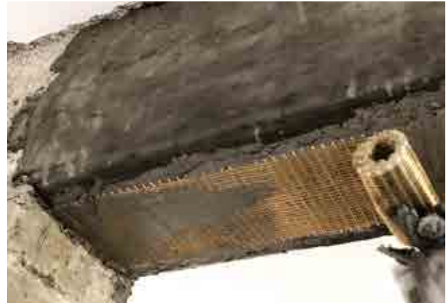
Flexural strengthening.
