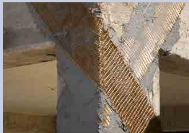
Strengthening to absorb the action exerted by an infill wall.
