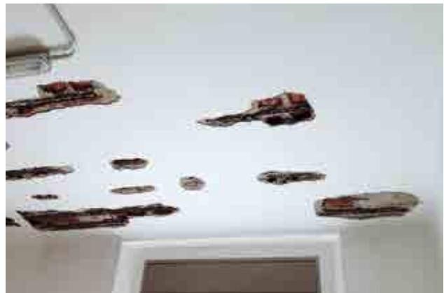
The phenomenon of shatter and falling of ceiling fragments expands and evolves over time as the consequence of several different factors and requires timely intervention to render affected structures safe.
