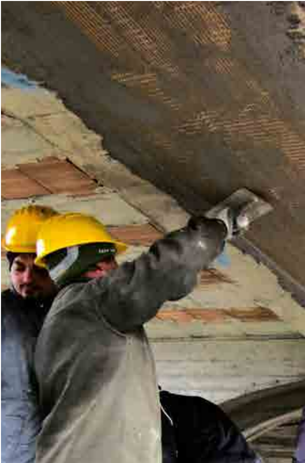
Flexural strengthening.
