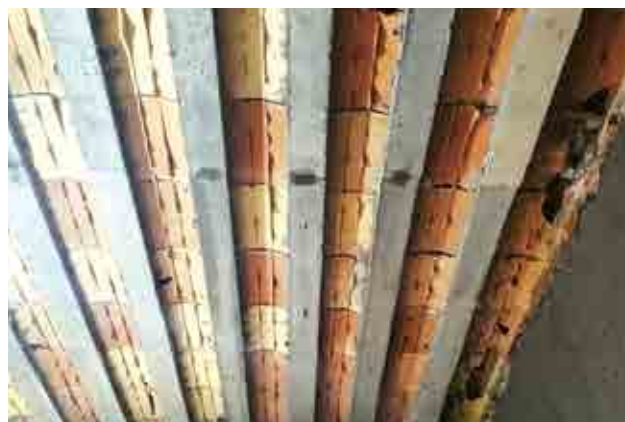
The second phase involves the geometric reconstruction of the joist using MX-R4 Repair structural repair mortar.
