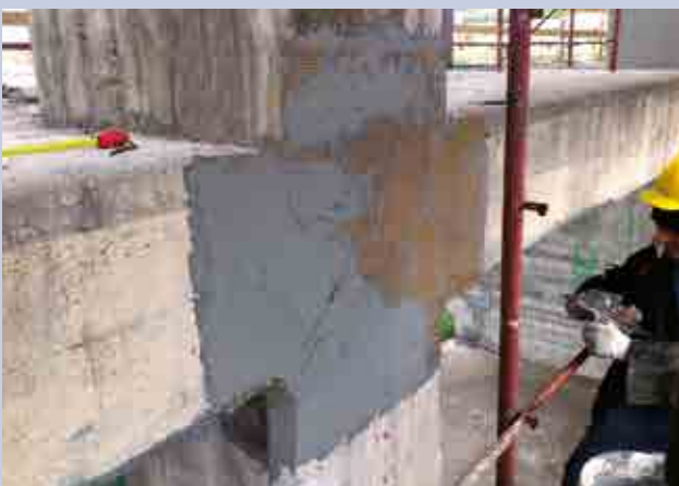
Increasing the shear resistance of the beam-column joint.
