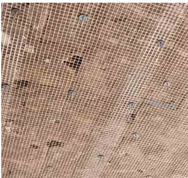
Installed SAFENET system
