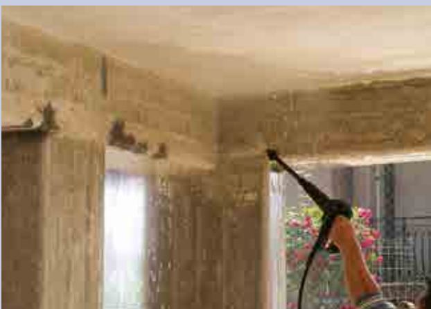
Saturating the support.
