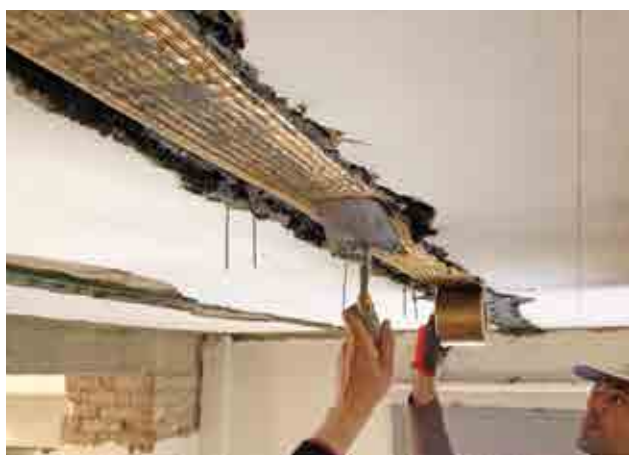
Applying the FRCM strengthening system.
